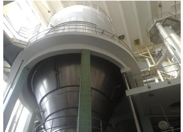
*Figure 2: Spray dryer at Schwarzwaldmilch with an evaporation capacity of up to 3000 kg per hour.*
